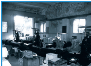
Supply and Installation of HSC Pumpset for 20 MGD Water Supply System
