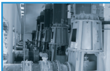
Installation of Vertical Turbine Pumpset for 125 MLD Drinking Water Supply Project
