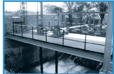
Engineering, Supply and Installation of VT Pumpset- River Water Pumping System
