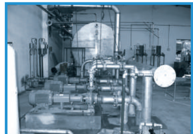
Supply and Installation of Hot Water Pumping System
