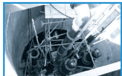
Supply and Installation of Submersible Pumpsets- 110kw & 180kw
